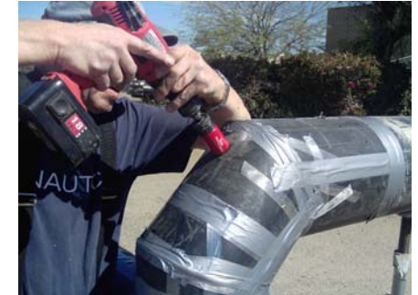
Drill min. 1" Hole on top side of center cover
