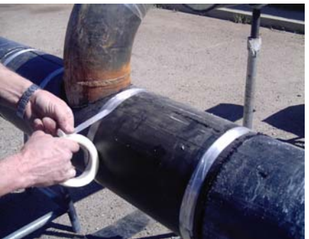
Seal all seams using Duct tape
