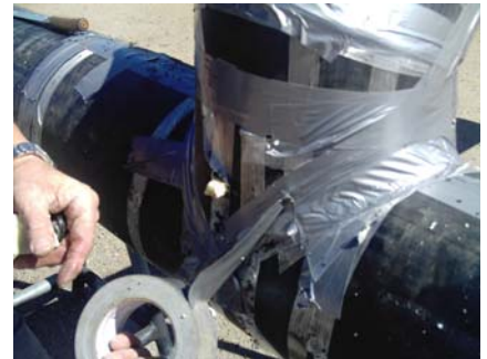
Seal once foam begins to escape
