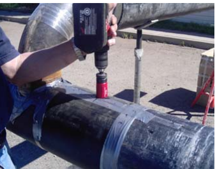
Seal all seams using Duct tape
