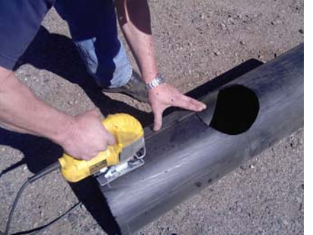
Split the jacket to slip on pipe
