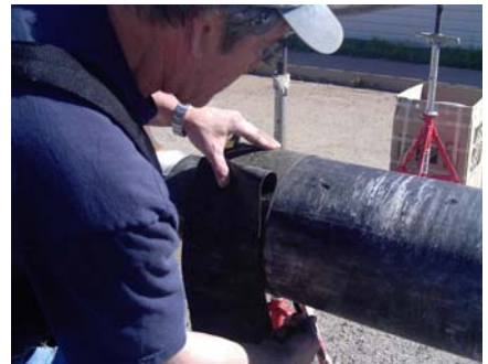
Draw a line for the jacket to be removed
