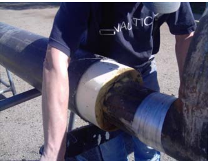
Remove the jacket on both cuts
