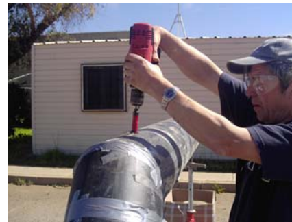
Drill min. 1/2" Hole on top side of 90
