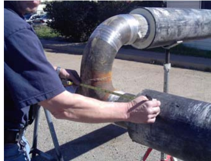
Mark the corresponding dimensions on pipe
