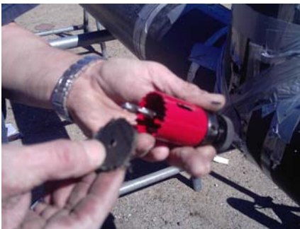
Save 1" slug to put back in hole after foaming
