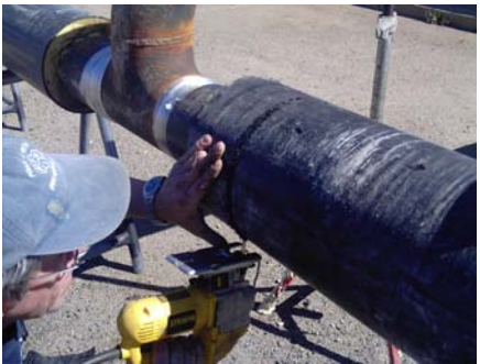
Cut the jacket on both sides of tee
