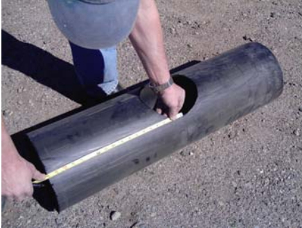
Measure center to end of sleeve
