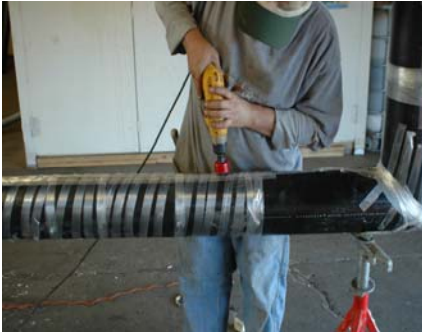
Drill 1" hole on each end of joint
