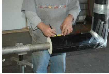
Measure sleeve length and mark jacket on both sides
