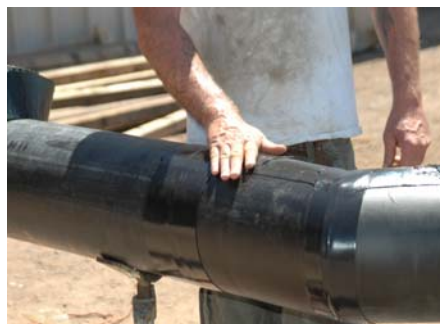
Mix equal parts of A & B and pour in joint. Remove tape and apply heat shrink to all seams
