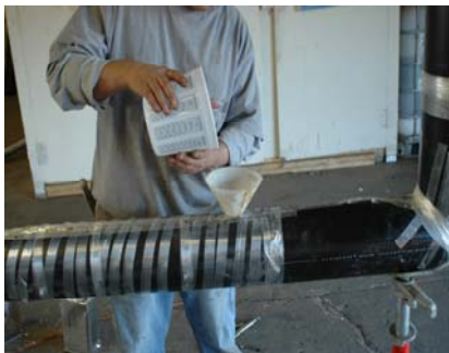
Mix equal parts of A & B and pour in joint. Remove tape and apply heat shrink to all seams
