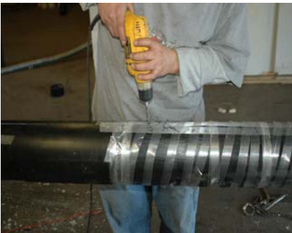
Drill 1" hole on each end of joint
