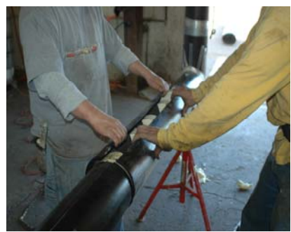
Install HDPE sleeve
