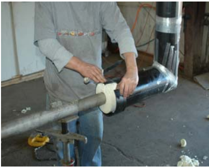
Cut jacket to expose foam (approx. 3") on both ends of joint
