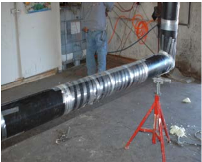
Tape sleeve to hold and seal for foam
