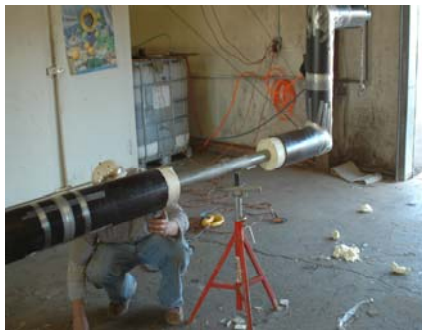
Cut jacket to expose foam (approx. 3") on both ends of joint
