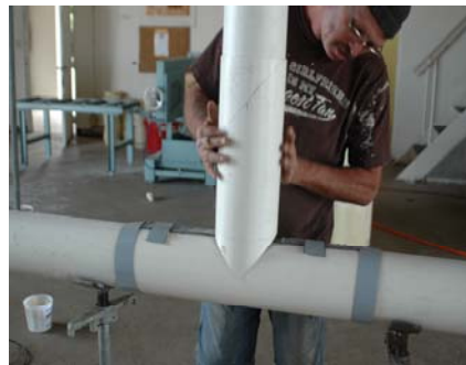
Slide branch sleeve into position
