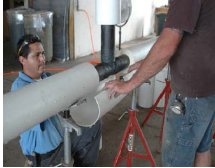
Install pre-drilled sleeve on pipe
