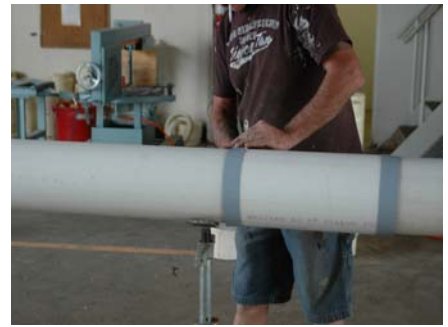
Apply tapecoat to all seams
