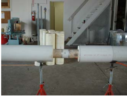
With pipe connected installed slide sleeve
