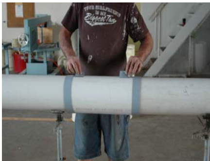
Apply tapecoat over 1" hole
