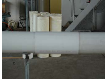
into position on pipe
