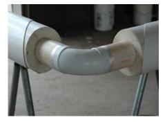
With fitting installed slide sleeve
