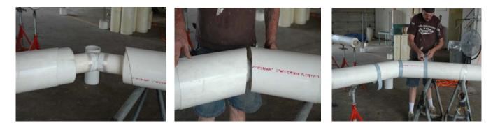
With fitting installed slide sleeve
