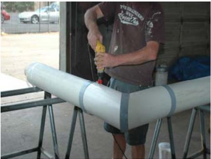
**Drill 1" hole on each side for foam**
