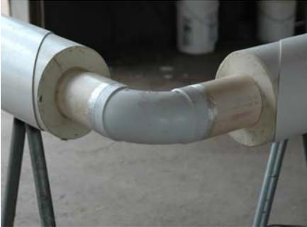
**With fitting installed slide sleeve**
