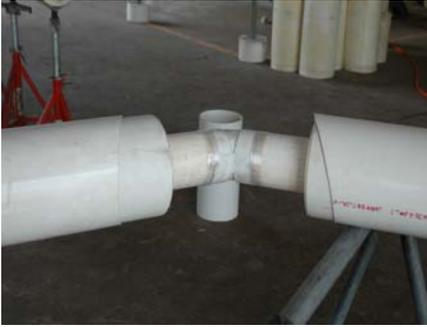
**With fitting installed slide sleeve**
